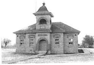
Fairfield School House, 1898
