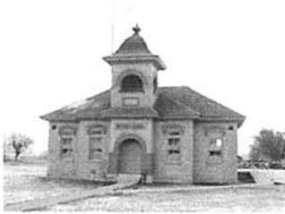
Fairfield School House, 1898
